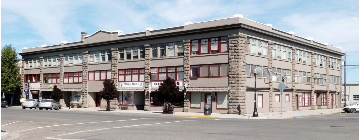
Mercantile and Milling Company Building, Enterprise
